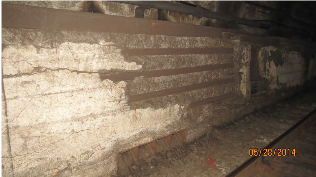
Photo E20: Cracked, Delaminated Concrete adjacent to Severe Spall with exposed steel on North Bench Wall, Line 2 Station 90+38. Total deficient area was 18' long x full height x up to 16" deep locally, near manhole niche. Photo Ref. GK12-029, looking Begin, North.
