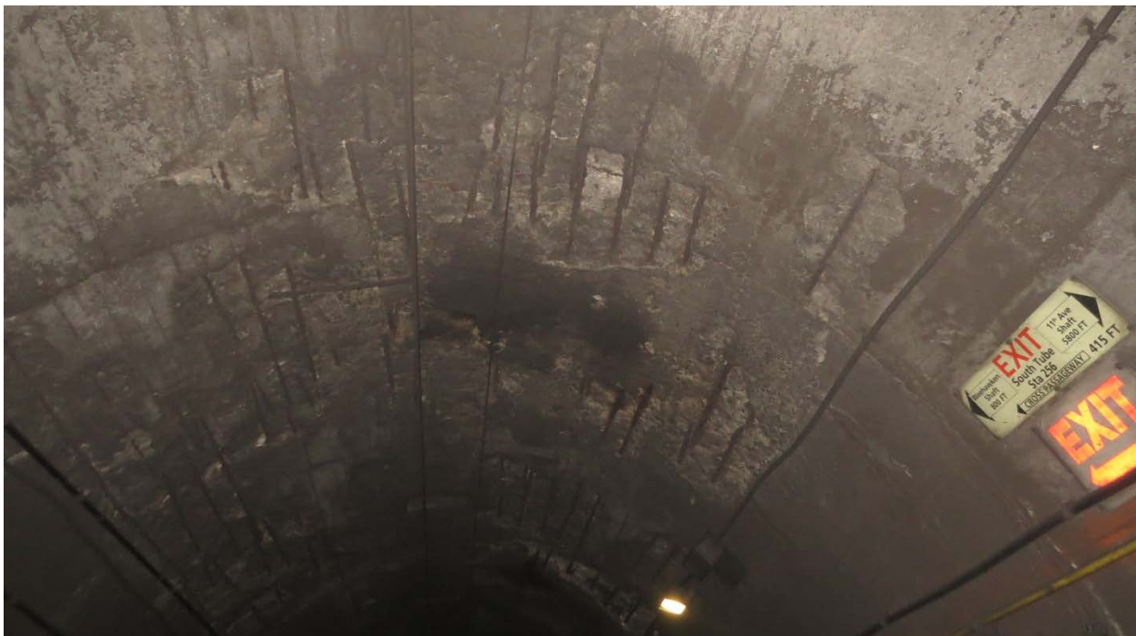
Photo N12: Several Severe Spalls up to 4" deep with exposed rebar over a 37' length of the South Tube. Spalls occur between the 10:00 and 2:00 positions on the South and North Walls, beginning near South Tube Station 256+00. Photo Ref. GK05-060, looking End, Up.
