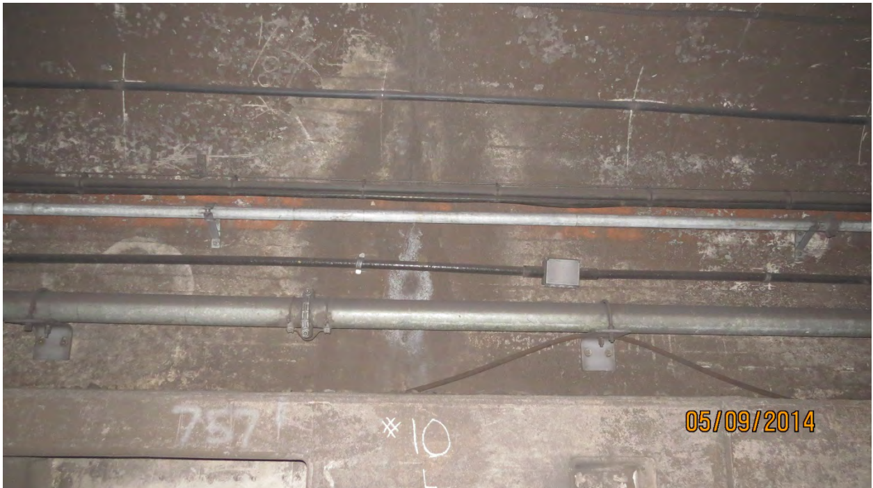
Photo N20: Light Efflorescence along transverse joint, on South Wall at South Tube Station 233+13. Photo Ref. GK04-046, looking South.
