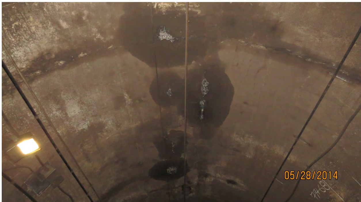
Photo E19: Efflorescence, Damp Incrustation, and Active Moisture along longitudinal joints near Crown, South and North Walls, Line 2 Station 79+68. Photo Ref. GK12-049, looking End, Up.
