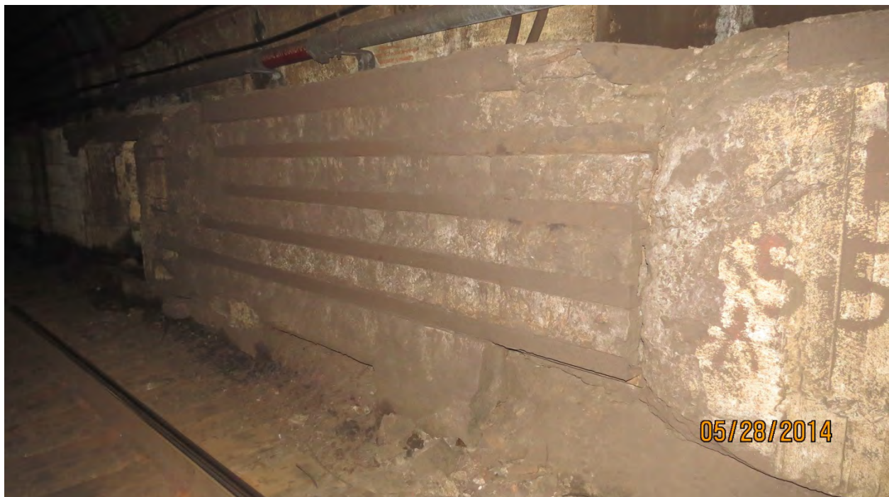
Photo E13: Full-Height Severe Spall with exposed steel extending between manhole refuge niches, North Bench Wall near Line 2 Station 82+14. No steel plates were installed to cover missing concrete along top of bench. Photo Ref. GK12-042, looking End, North.
