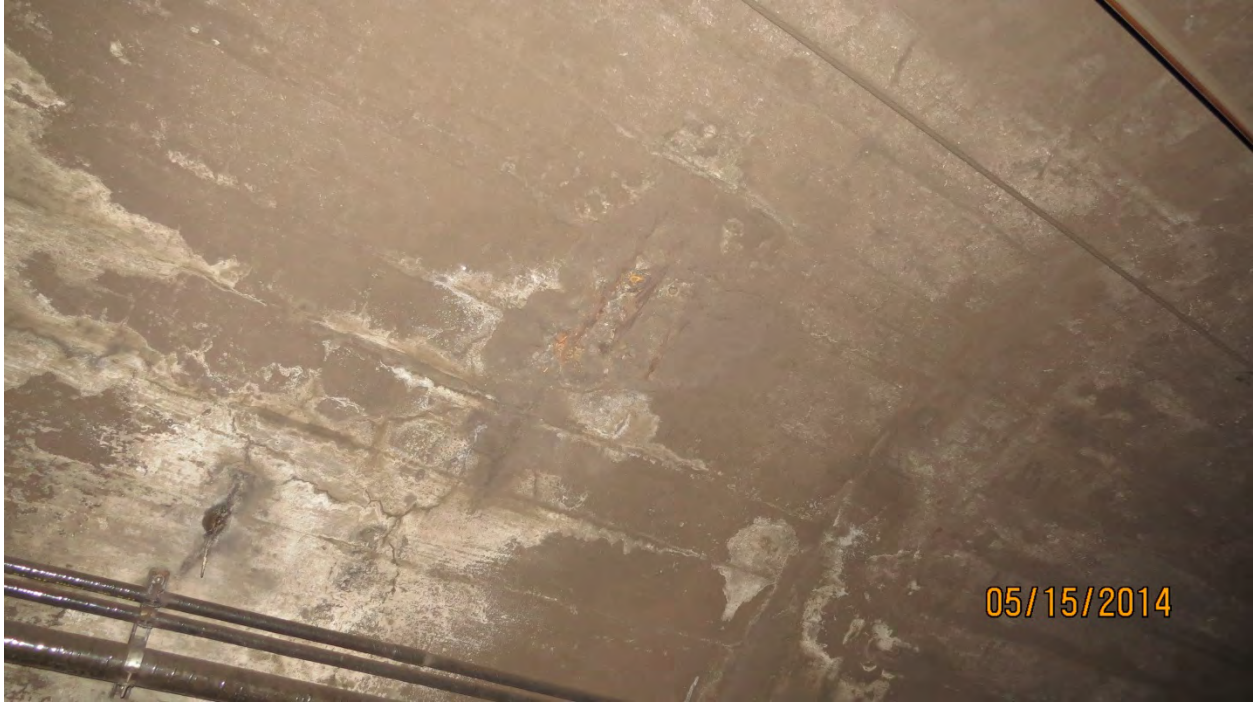
Photo E10: Severe Spall 6' long x 12" wide x 1" deep at 10:15 position with exposed steel, North Wall, Line 1 Station 104+38. Stalactite and point of Active Moisture also visible. Photo Ref. GK08-067, looking Begin, North.
