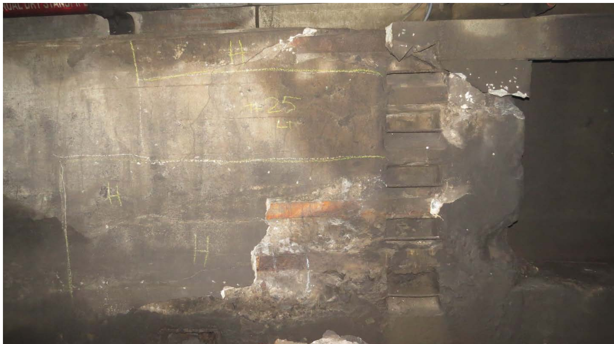
Photo N18: Delaminated Concrete area, 40 square feet, and Severe Spalls with exposed steel on South Bench Wall, 4' long x 3' high x 3-1/2" deep and 2-1/2' L x 1' high x up to 6" deep, at South Tube Station 241+03. Photo Ref. GK05-020, looking South.
