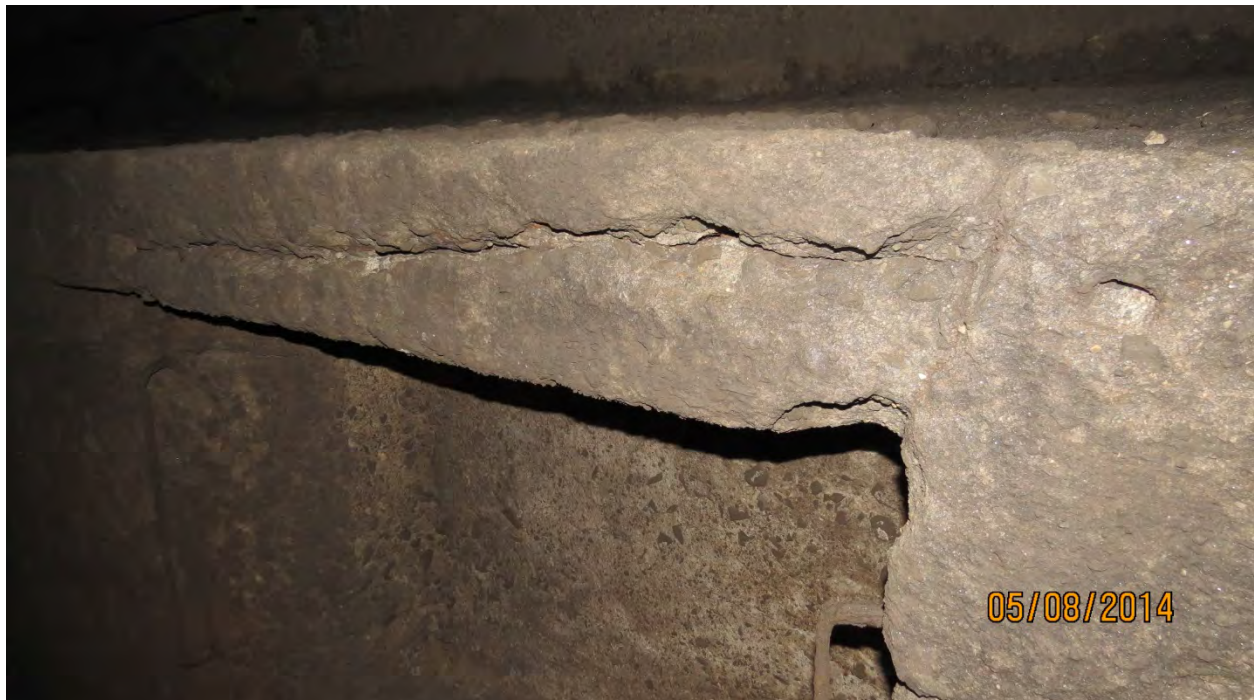
Photo N6: Longitudinal Severe Crack 5' long x up to 5/16" wide between manhole refuge niche and Top of Bench, North Bench Wall, North Tube Station 233+36. Photo Ref. GK03-047, looking End, North.
