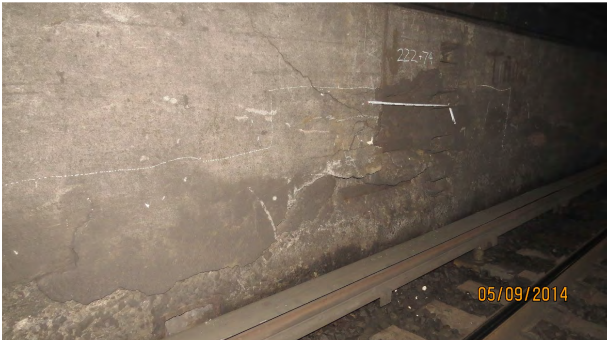
Photo N16: Delaminated Concrete 21' long x 3' to 4-1/2' high and a Severe Spall 5' long x 3' high x up to 4-1/2" deep on North Bench Wall near South Tube Station 222+54. Photo Ref. GK04-006, looking Begin, North.
