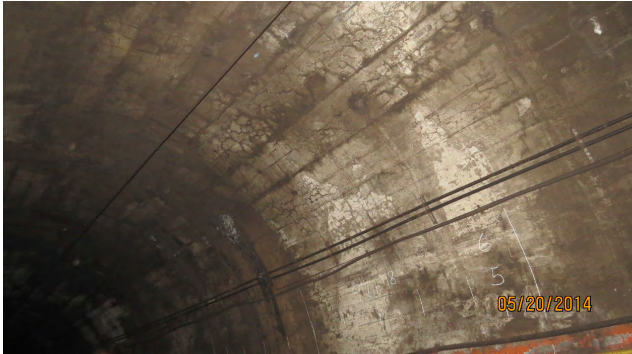
Photo E6: Map Cracking, with cracks up to 1/32", North Wall, Line 1 Station 97+78. Incrustation with Efflorescence and Active Moisture visible in background, at Line 1 Station 97+85. Photo Ref. GK11-083, looking End, North.
