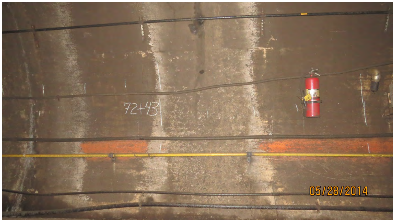
Photo E21: Honeycombing over an area 4' long x 5' wide adjacent to top of bench, South Wall, Line 2 Station 72+43. Photo Ref. GK12-072, looking South.
