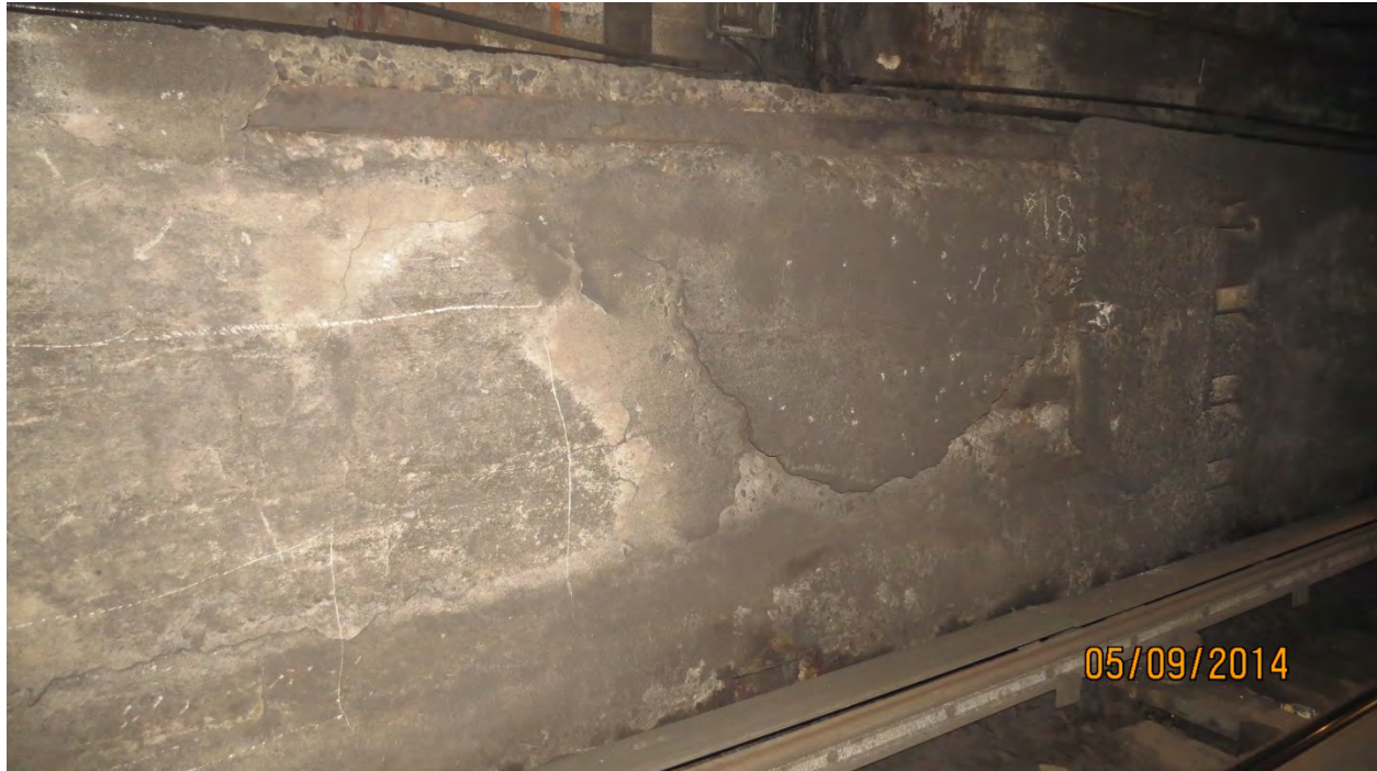
Photo N17: Delaminated Concrete area, 20 square feet, and Severe Spalls with exposed steel, 10' long x 1' high x up to 5-1/2' deep and 6' long x 3' high x 4" deep on North Bench Wall near South Tube Station 238+50. Photo Ref. GK04-077, looking Begin, North.
