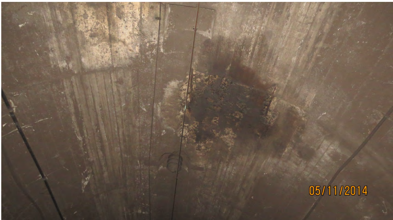
Photo N8: Two Severe Spalls with exposed rebar, 7' long x 1' wide x 4" to 5" deep and 2' long x 1' wide x 4" deep, near Crown, with adjacent Honeycombing and Active Moisture. South Wall, North Tube Station 251+75. Photo Ref. GK06-042, looking Begin, Up.
