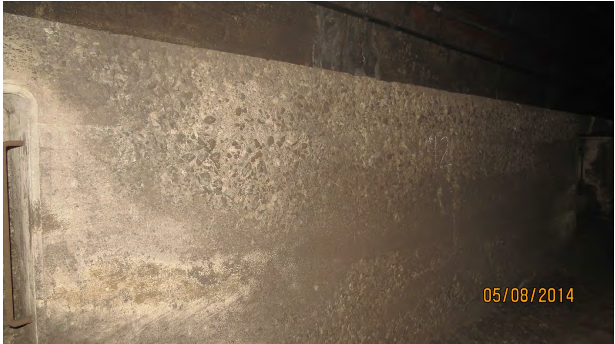
Photo N25: Honeycombing over approximately 60% of surface area of bench wall between adjacent manhole refuge niches. North Bench Wall, near North Tube Station 230+24. Photo Ref. GK03-029, looking Begin, North.
