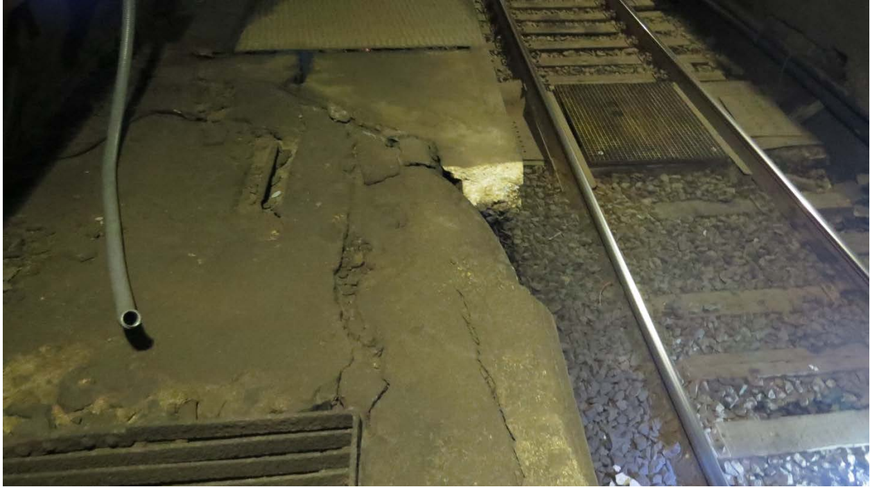
Photo N19: Cracked, Spalled Concrete on Top of Bench above location with Severe Spalls, South Bench Wall near South Tube Station 241+03. Up to 6" of concrete is missing, and top surface is severely cracked. Photo Ref. GK05-023, looking End, Down.
