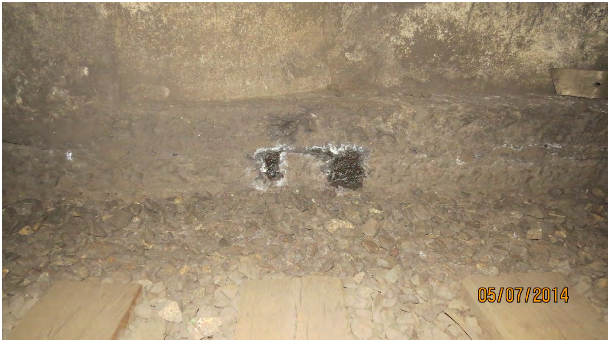
Photo N4: Short longitudinal Moderate Crack with efflorescence and Active Moisture with inflow of a few drops per minute. Crack is located near bottom of North Bench Wall, North Tube Station 224+66. Photo Ref. GK02-027, looking North.
