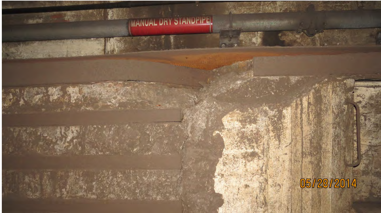
Photo E12: Typical Severe Spall with exposed steel adjacent to manhole refuge niche, North Bench Wall near Line 2 Station 86+14. A steel plate was installed to cover missing concrete along the top of bench walking surface. Photo Ref. GK12-039, looking North.
