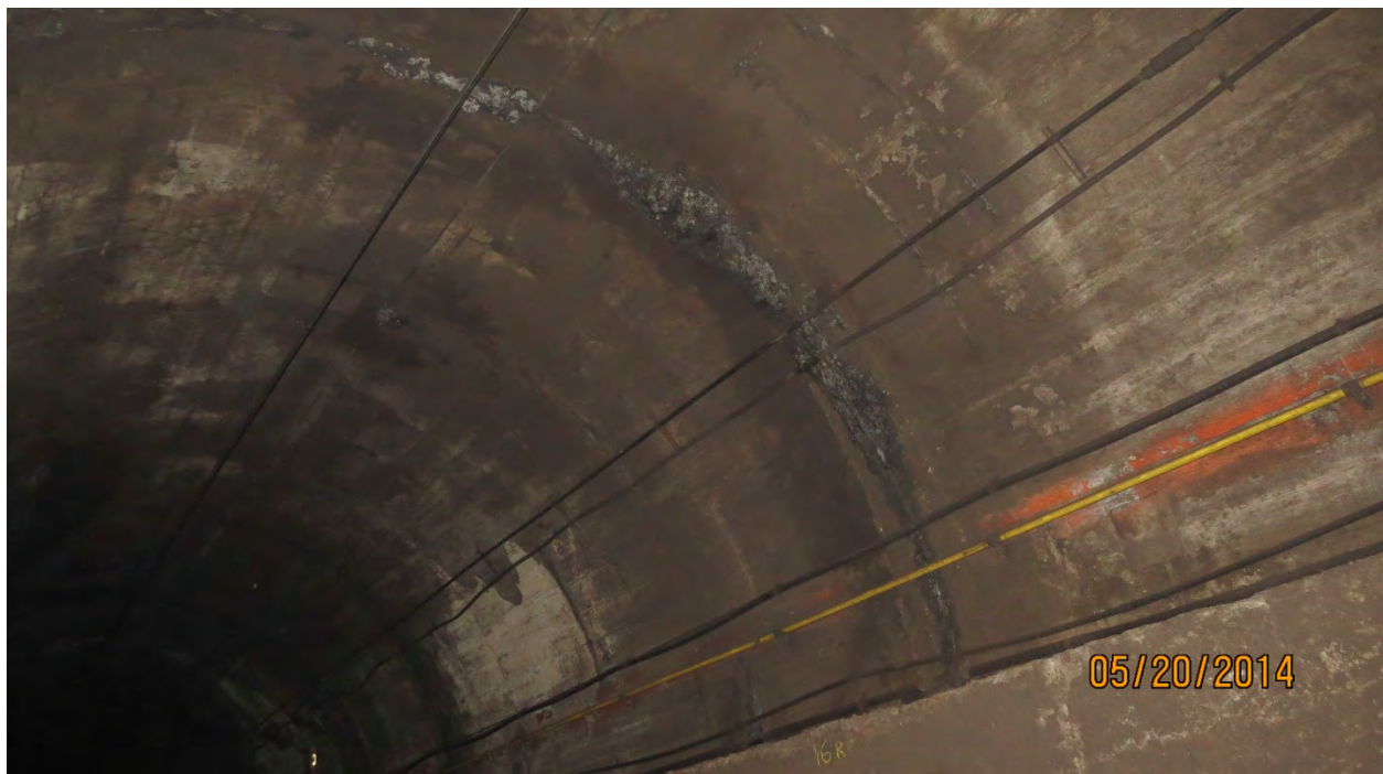
Photo E17: Efflorescence, Damp Incrustation, and Active Moisture along transverse joint, North Wall, Line 1 Station 95+29. Photo Ref. GK11-071, looking End, North.
