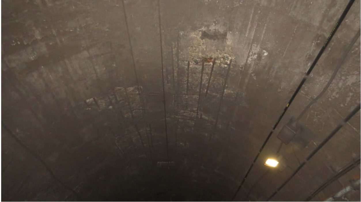
Photo N13: Severe Spalls up to 4" deep with exposed rebar between 10:00 and 2:00 positions on South and North Walls over a 50' length of South Tube. A 1' x 1' area near South Tube Station 256+80 was a locally deep Void/Hole. Photo Ref. GK05-067, looking Begin, Up.
