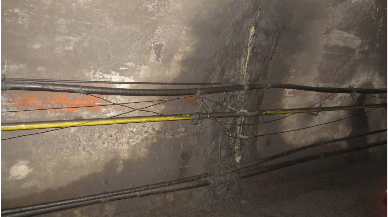
Photo N23: Wet Incrustation and Active Moisture below 2:00 position, with leakage of several drops per minute. Incrustation 3" to 4" thick was observed on wall and top of bench. North Wall, South Tube Station 238+67. Photo Ref. GK05-009, looking Begin, North.
