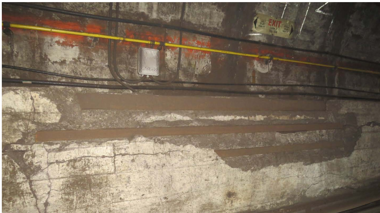
Photo E15: Severe Spall with exposed steel at Splicing Vault, South Bench Wall near Line 2 Station 103+99. Photo Ref. BBS1 IMG_0028, looking End, South.
