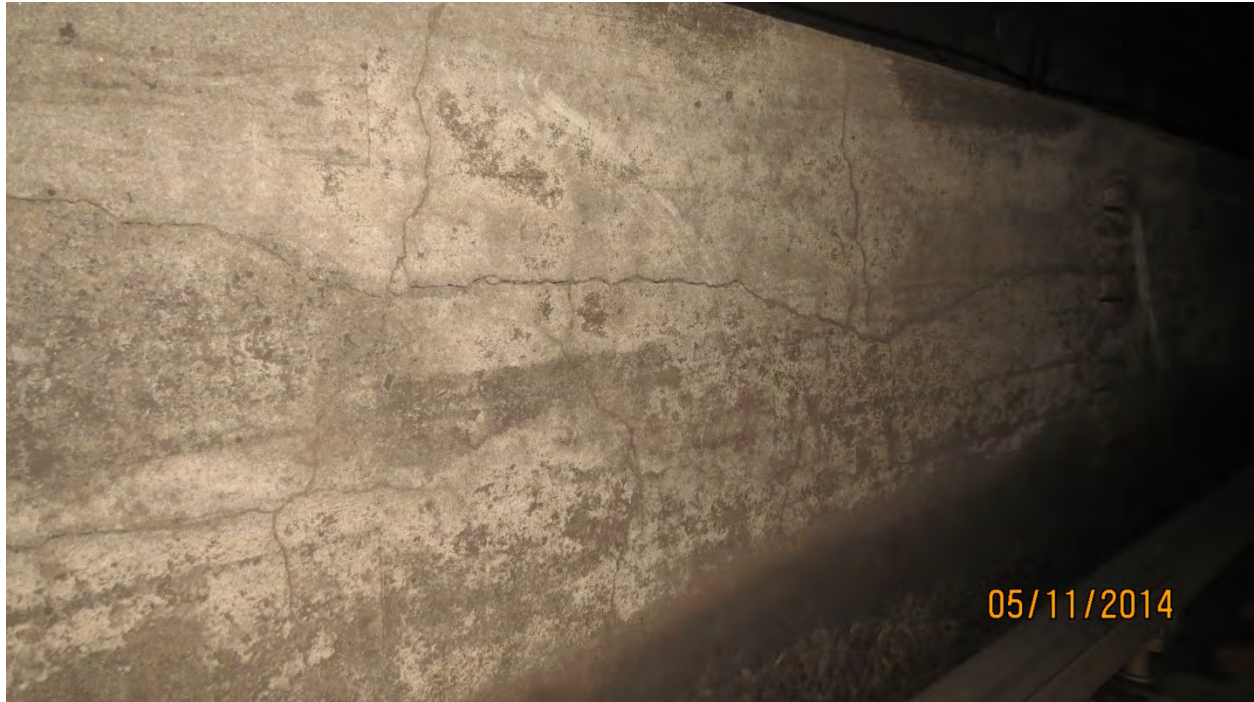
Photo N5: Longitudinal crack up to 3/16" wide and scattered transverse cracks up to 1/16" wide, South Bench Wall, North Tube Station 246+81. Damp concrete on lower 2' to 3' of wall and honeycombing on lower 1' to 2' of wall. Photo Ref. GK06-034, looking End, South.
