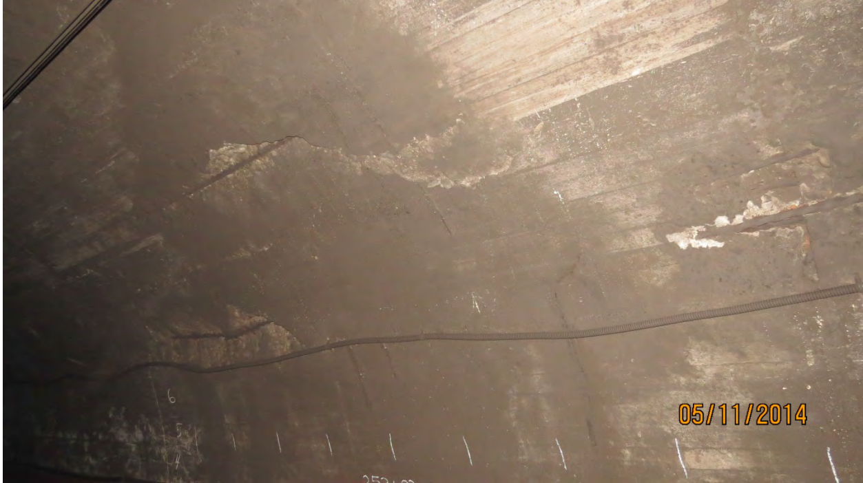
Photo N9: Three 4" deep Severe Spalls with exposed rebar, 6' long x 2' wide, 4-1/2' long x 1' wide and 3' long x 2' wide, on South Wall near North Tube Station 252+82. Delaminated Concrete 18' long x 5' wide between spalls. Photo Ref. GK06-047, looking Begin, South.
