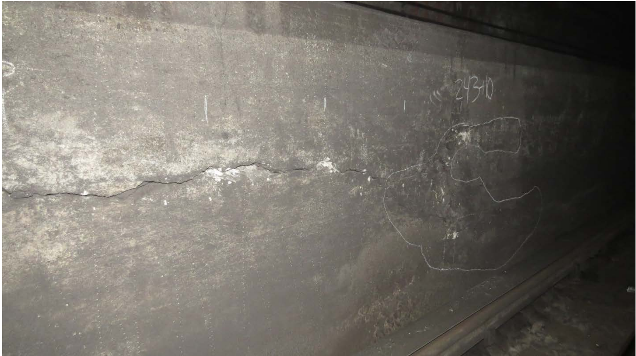
Photo N7: Longitudinal Severe Crack 110' long x up to 1/4" wide with scattered Moderate Spalls along crack and Concrete Delamination 8' long x 4' high near Station 243+10. North Bench Wall, South Tube Station 243+20. Photo Ref. GK05-035, looking Begin, North.
