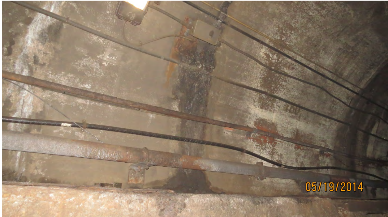
Photo E16: Efflorescence, Damp Incrustation, and Active Moisture along transverse joint, North Wall, Line 2 Station 91+50. Moderate buildup of incrustation on wall and top of bench. Photo Ref. GK10-079, looking Begin, North.
