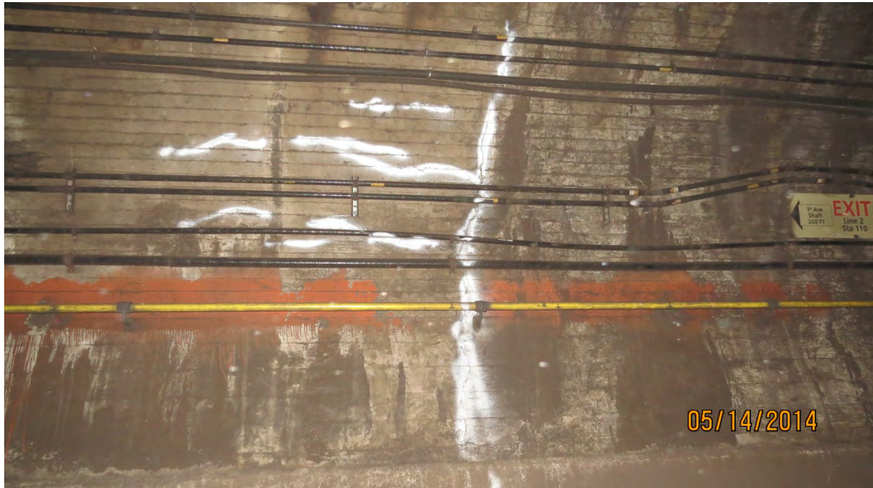
Photo E1: Typical Transverse Moderate Crack up to 1/16" wide, South Wall, Line 2 Station 109+90. Photo Ref. GK07-020, looking South.
