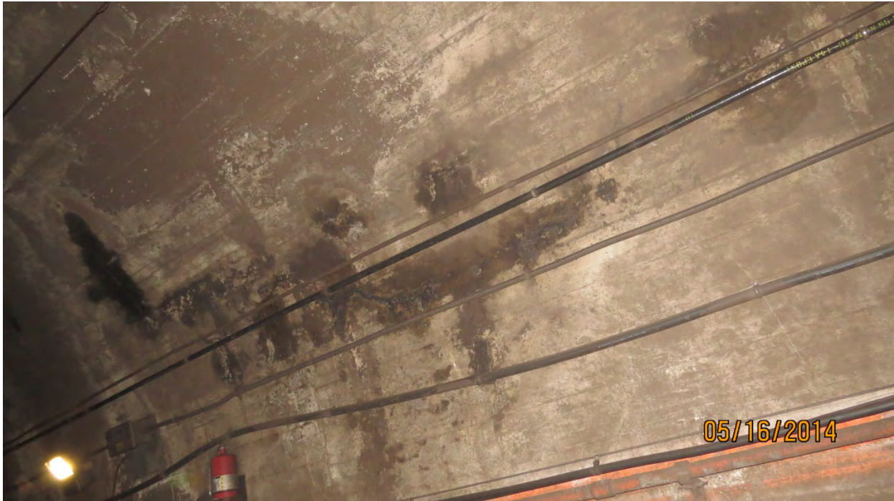
Photo E4: Longitudinal Moderate Crack up to 1/16" wide Staining, Efflorescence and Active Moisture, South Wall, Line 1 Station 88+26. Photo Ref. GK09-033, looking Begin, South.
