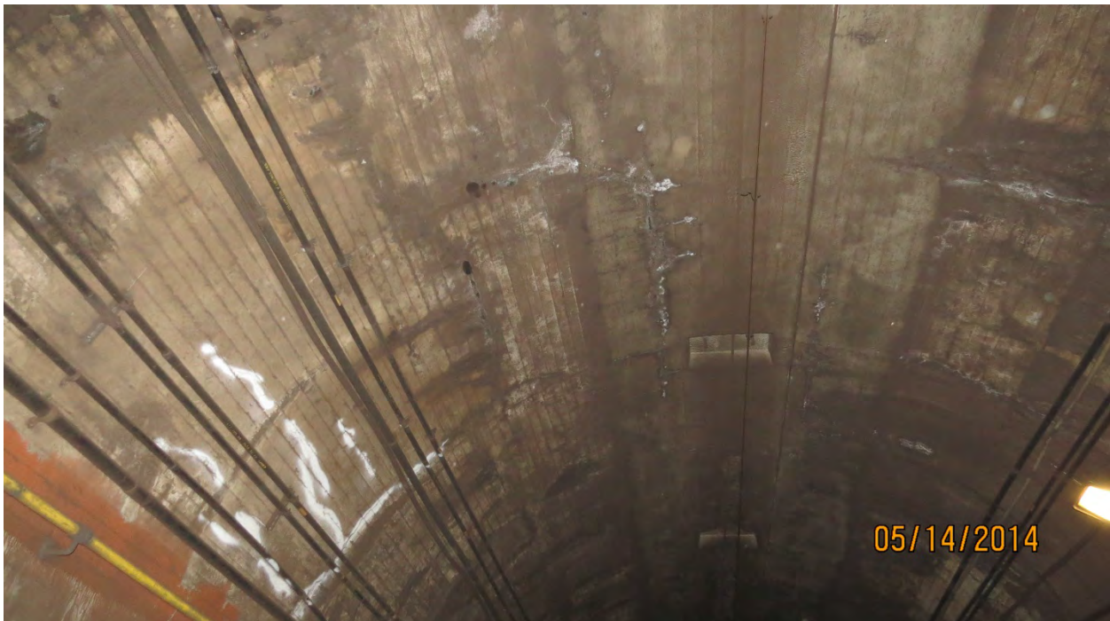
Photo E3: Longitudinal Moderate Crack with Efflorescence near Crown. Isolated Damp Spots with Active Moisture on South Wall, Line 2 Station 109+90. Photo Ref. GK07-023, looking End, Up.
