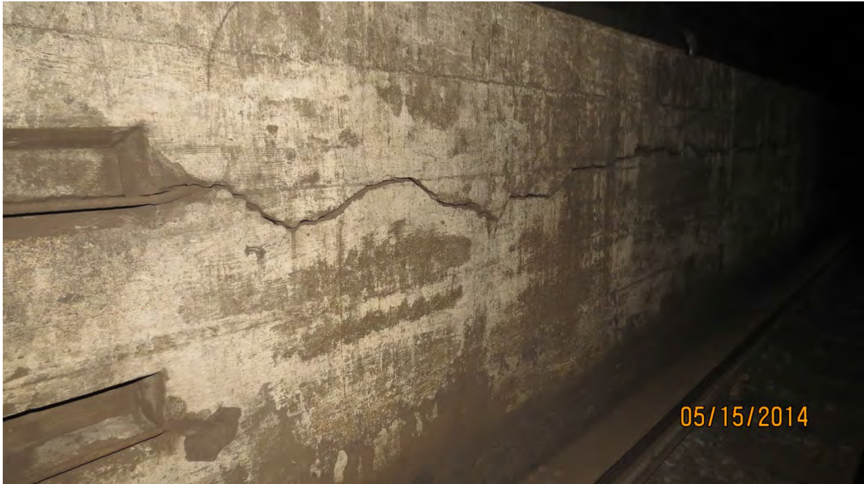
Photo E8: Longitudinal Severe Crack 25' long x up to 3/4" wide, North Bench Wall, Line 1 Station 105+20. Photo Ref. GK08-058, looking Begin, North.
