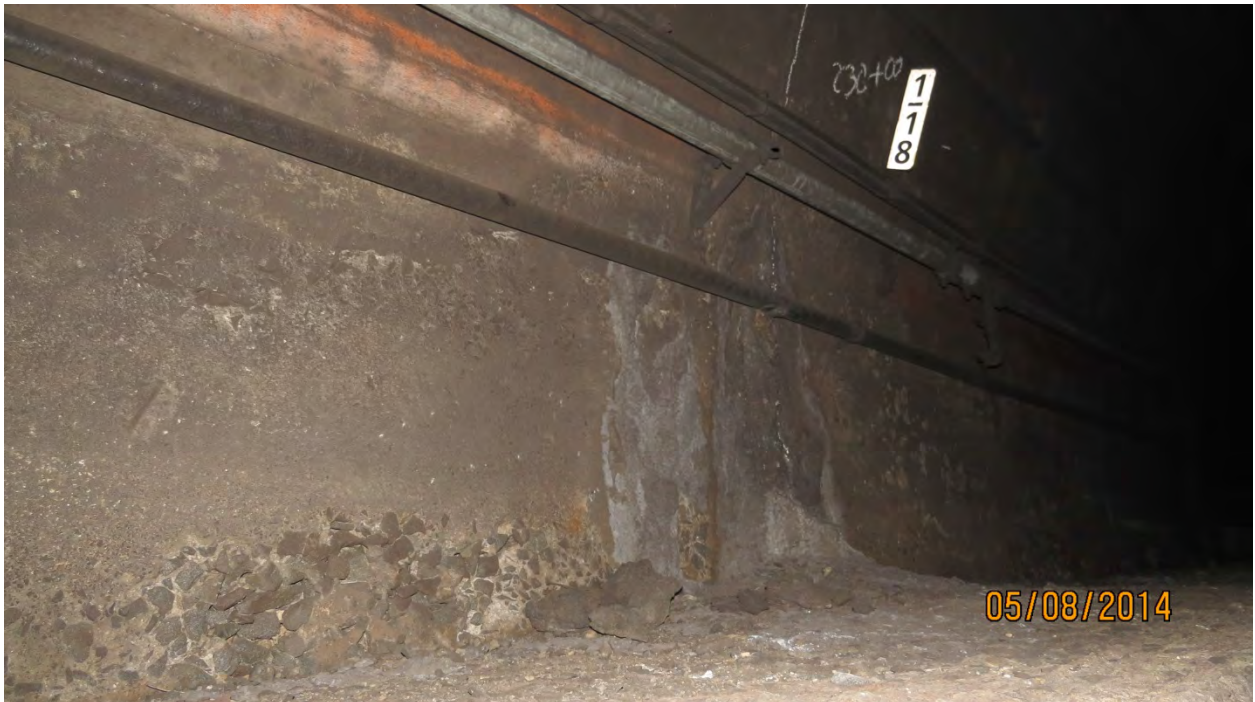
Photo N24: Honeycombing 3' long x 1' wide on wall along top of bench, North Wall, near North Tube Station 230+24. Photo Ref. GK03-028, looking Begin, North.
