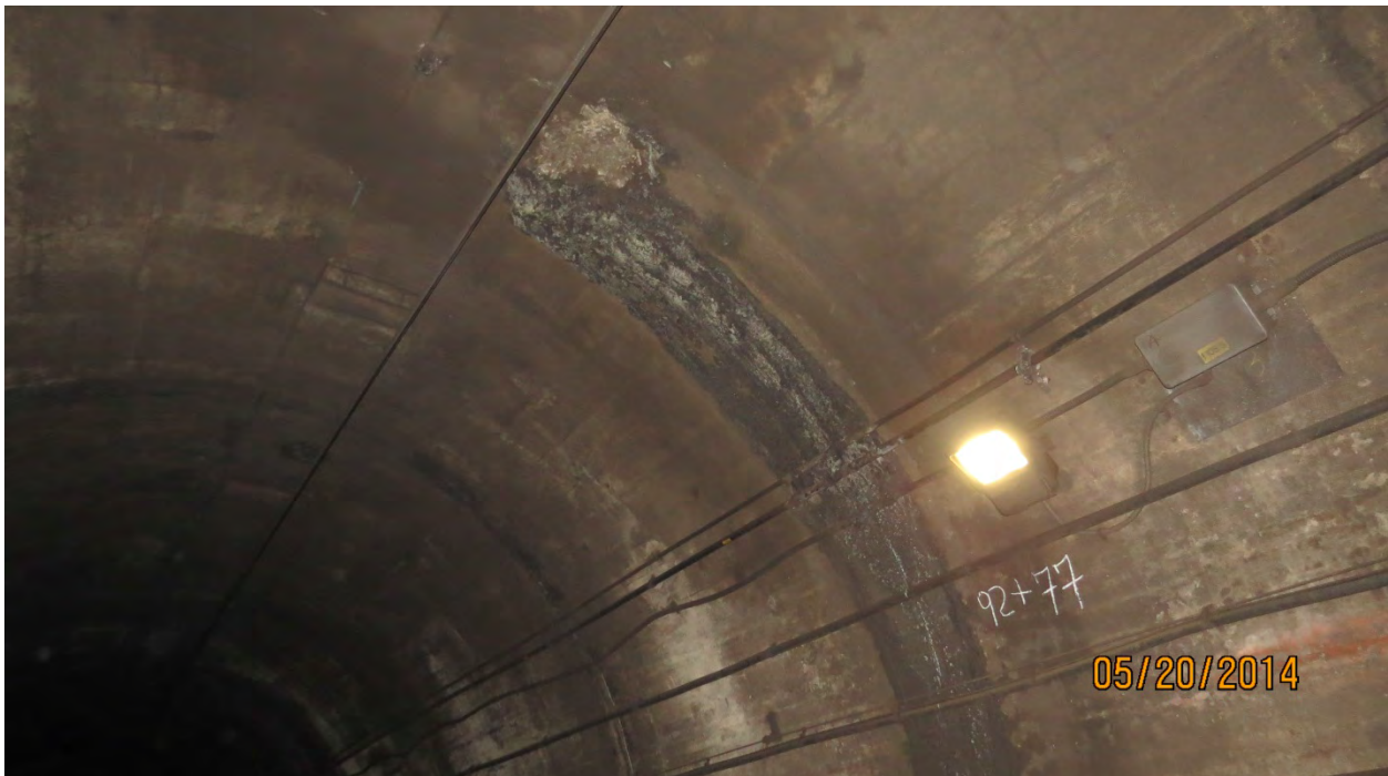
Photo E9: Severe Spall 2' long x 1.5' wide x up to 4" to 5" deep near Crown, South Wall, Line 1 Station 92+77. Incrustation, Stalactites, Efflorescence and Active Moisture with inflow of 15 drops per minute adjacent to Spall. Photo Ref. GK11-055, looking Begin, South.
