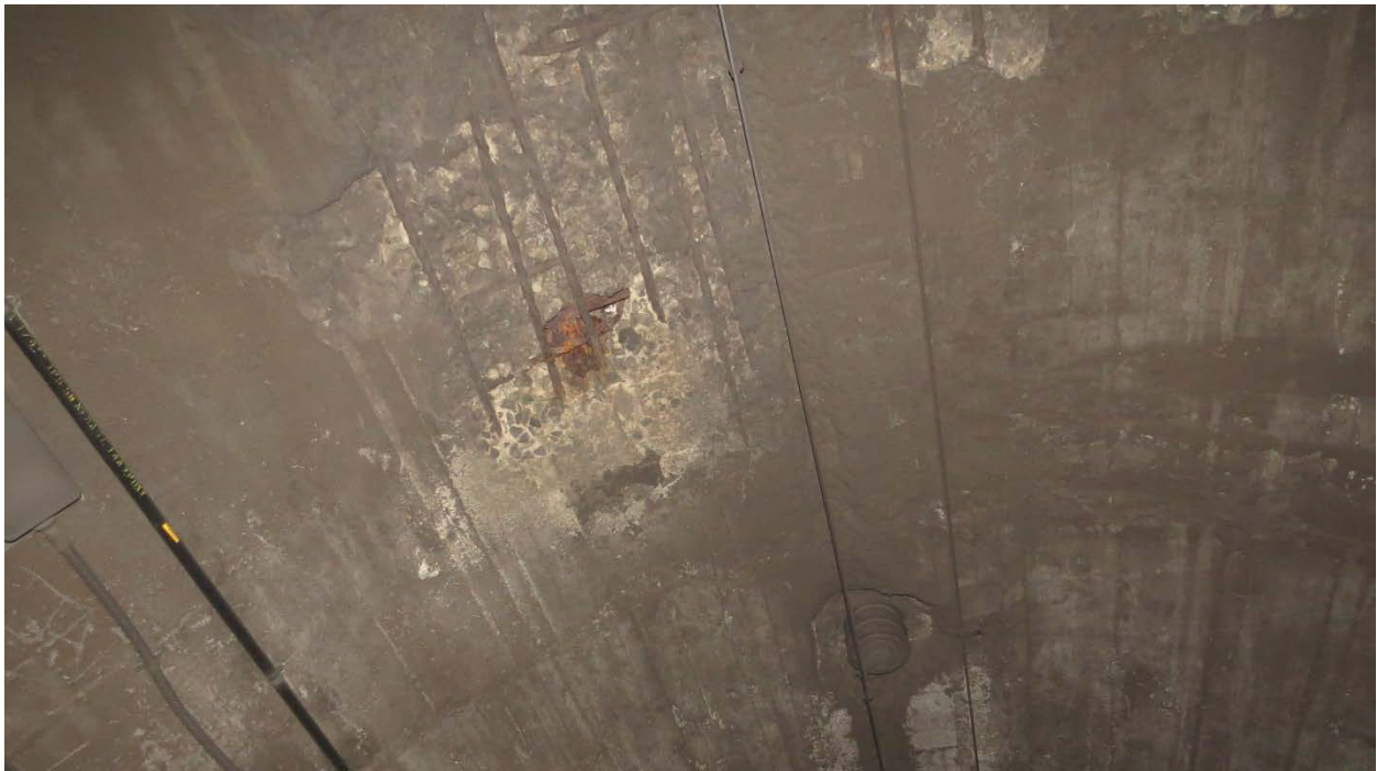
Photo N14: Close-Up of 4" deep Severe Spall with exposed rebar and 1' long x 1' wide locally deep Void/Hole in concrete lining, South Wall, near South Tube Station 256+80. Photo Ref. GK05-065, looking End, South, Up.
