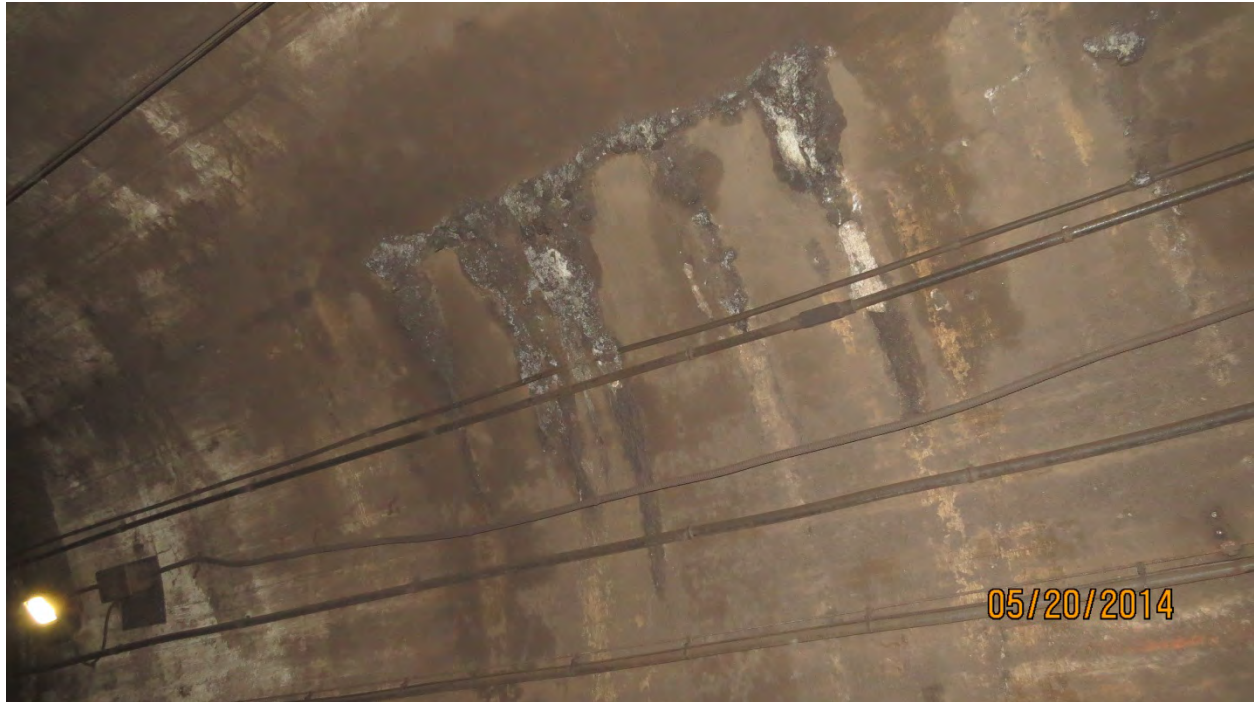
Photo E18: Efflorescence, Damp Incrustation, and Active Moisture along longitudinal joint, South Wall, Line 1 Station 95+45. Photo Ref. GK11-078, looking Begin, South.
