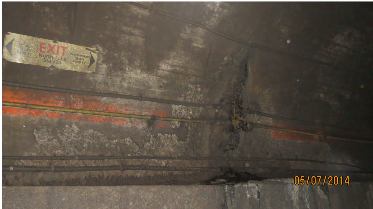
Photo N21: Incrustation and Active Moisture between 9:00 and 10:00 positions, South Wall at North Tube Station 220+09. Incrustation up to 7" deep on wall, top of bench with moderate leakage of several drops per minute. Photo Ref. GK02-006, looking End, South.
