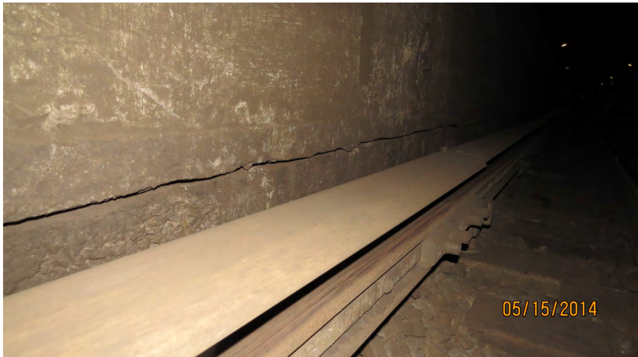
Photo E7: Longitudinal Severe Crack over 500' long x up to 1/2" wide near base of North Bench Wall, Line 1 Stations 100+00 to 105+20. Photo Ref. GK08-062, looking Begin, North.
