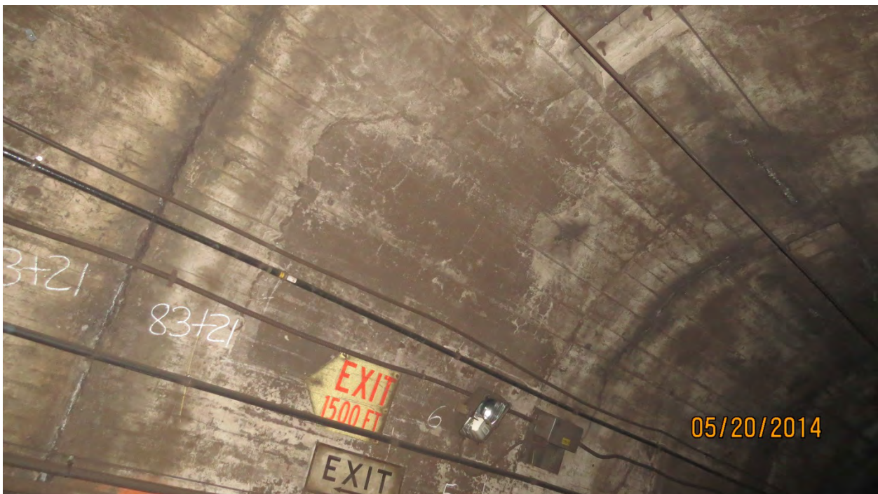
Photo E5: Diagonal Moderate Crack 6' long x up to 1/32" wide near Crown, transitioning to Transverse Moderate Crack, South Wall, Line 1 Station 83+21. Photo Ref. GK11-033, looking End, South.
