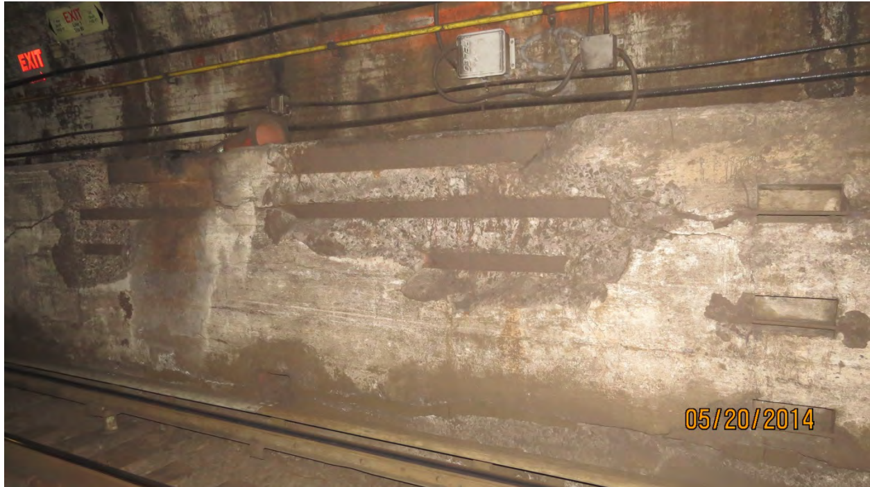
Photo E14: Severe Spall with exposed steel at Splicing Vault, North Bench Wall near Line 1 Station 79+87. Photo Ref. GK11-023, looking End, North.
