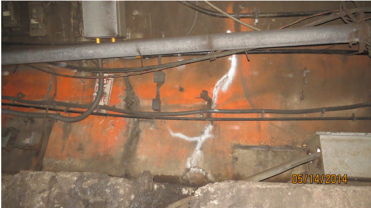
Photo E2: Transverse Moderate Crack up to 1/8" wide, North Wall, Line 2 Station 108+42. Photo Ref. GK07-045, looking Begin, North.
