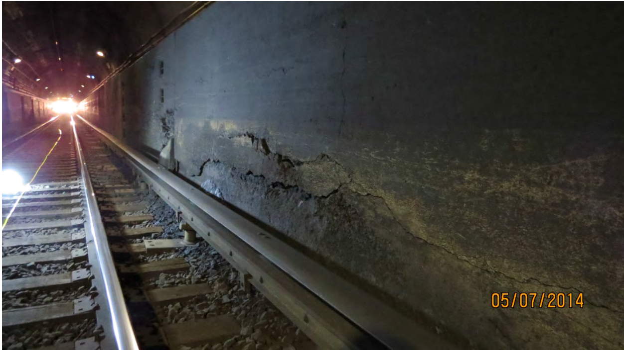
Photo N15: Longitudinal Severe Cracks, Delaminated Concrete 12' long x 3' high and localized Severe Spalls up to 4" deep in South Bench Wall near North Tube Station 222+64. Photo Ref. GK02-023, looking Begin, South.
