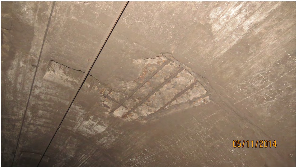
Photo N10: Severe Spall 6' long x 4' wide x 5" deep with exposed rebars on South Wall near North Tube Station 259+00. Areas of Concrete Delamination 6' long x 4' wide and 4' long x 3' wide adjacent to spall. Photo Ref. GK06-056, looking Begin, Up.
