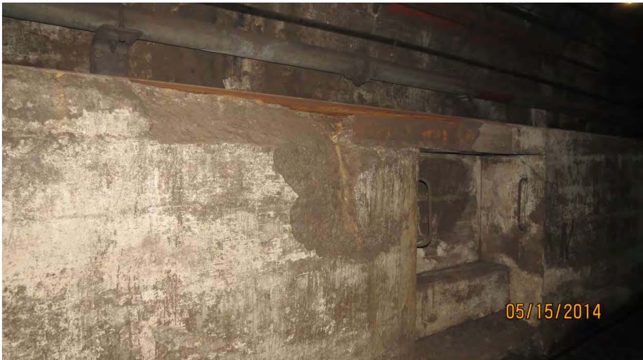
Photo E11: Typical Severe Spall with exposed steel adjacent to manhole refuge niche, South Bench Wall near Line 1 Station 100+77. A steel plate was installed to cover missing concrete along the top of bench walking surface. Photo Ref. GK08-081, looking End, South.
