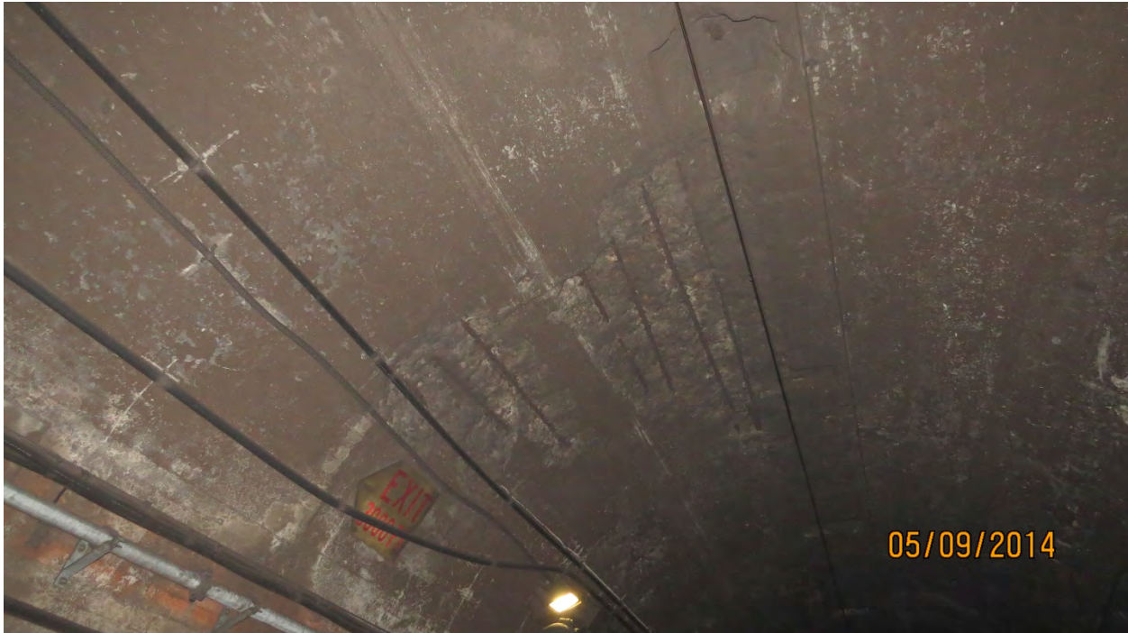
Photo N11: Two Severe Spalls with exposed rebar, 10' long x 4-1/2' wide x 4" to 5" deep and 6-1/2' long x 3' wide x 3" to 4" deep, on South Wall near South Tube Station 227+78. Photo Ref. GK04-020, looking End, Up.
