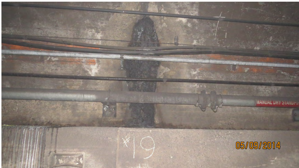
Photo N22: Damp incrustation up to 2" thick and minor Active Moisture along transverse joint below the 9:30 position on South Wall at South Tube Station 238+50. Photo Ref. GK04-080, looking South.
