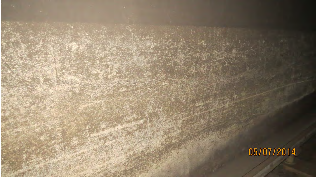
Photo N3: Longitudinal Moderate Crack up to 1/8" wide and Transverse Moderate Crack up to 1/16" wide, South Bench Wall, North Tube Station 225+42. Note the high water line from the inundation near top of image. Photo Ref. GK02-031, looking End, South.
