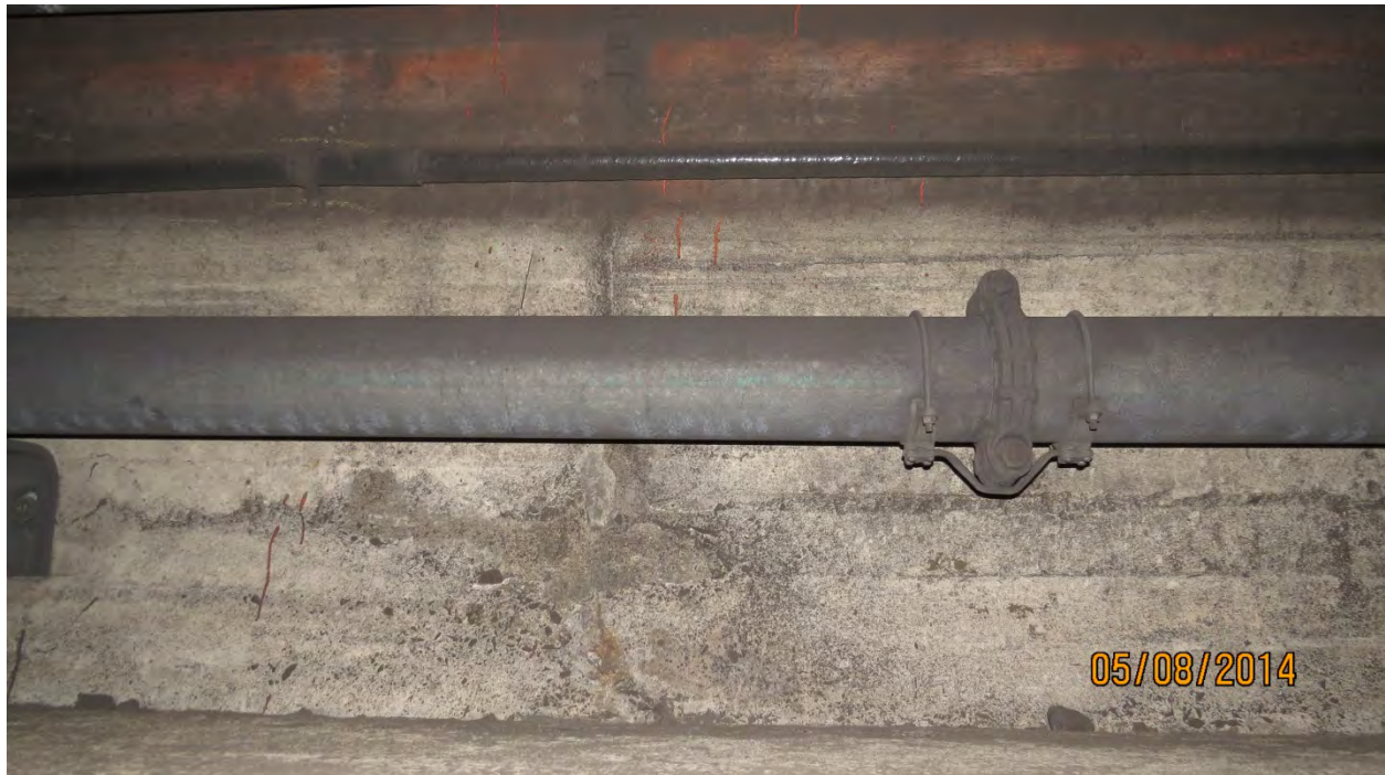
Photo N1: General View of Transverse Moderate Crack up to 1/16" wide on North Wall, North Tube Station 232+51. Photo Ref. GK03-036, looking North.
